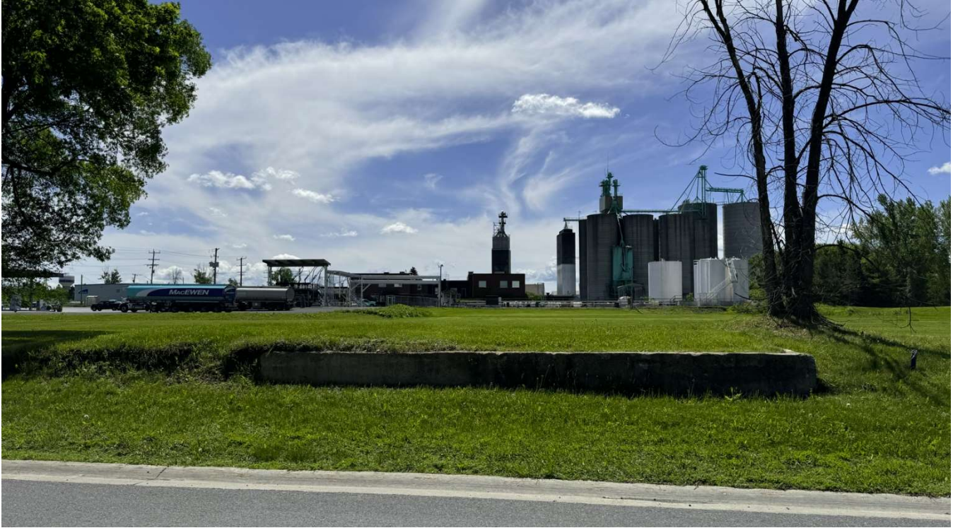
Exhibit G: Remnants of a building foundation along Mechanic Street West.
