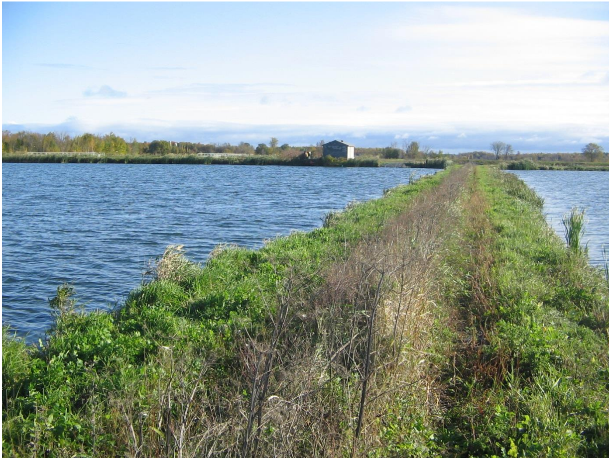
Figure 1-2– Alexandria Sewage Lagoon Facility
