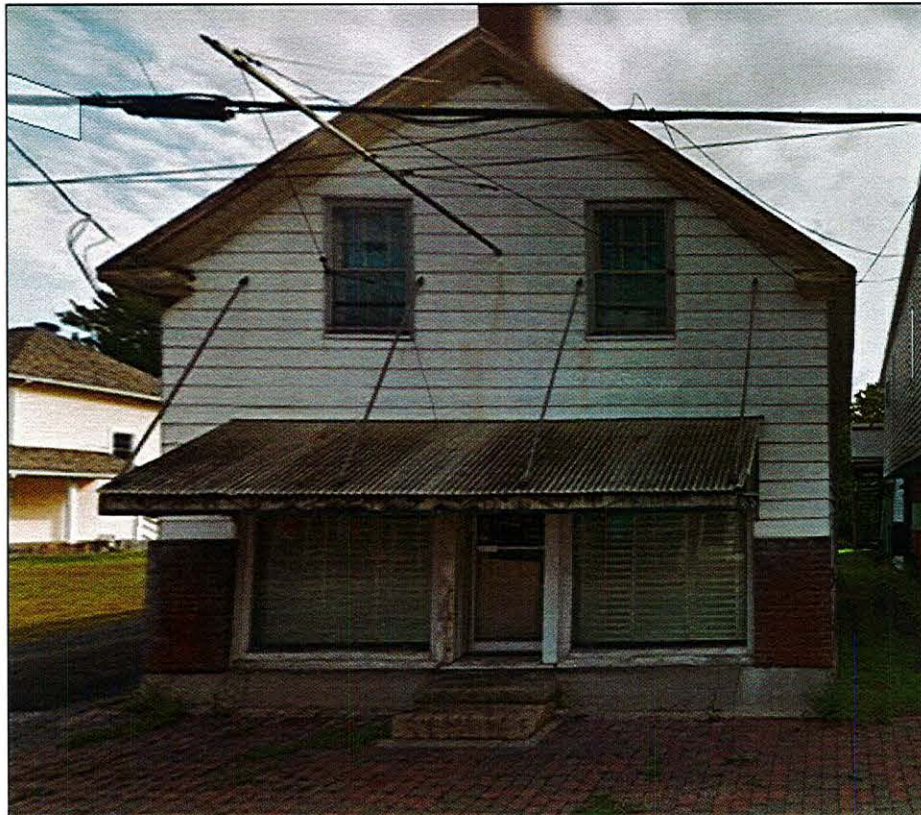
Building prior to renovations
