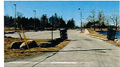
Figure 14: Existing entrance and gates to be shifted
