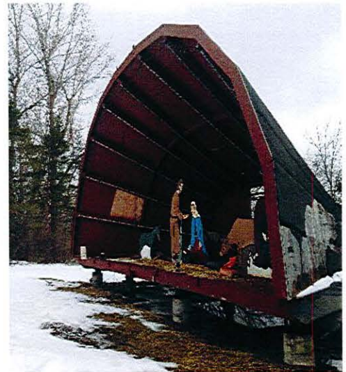
Figure 8: Existing band shell to be removed
