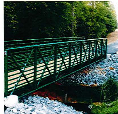
Figure 34: Prefabricated bridge example
