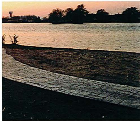
Figure 6: Existing unit pavers located by beach
