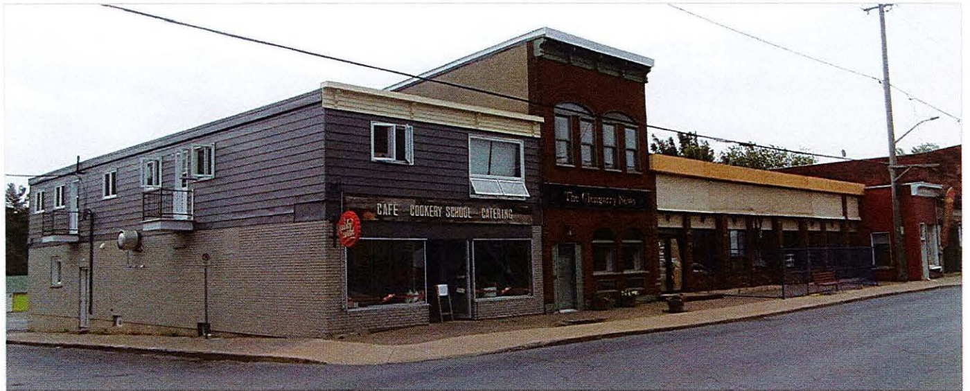
Current photo of the North Façade
