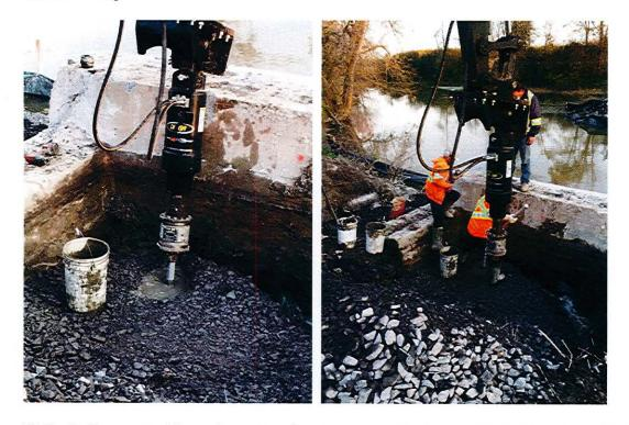
Helical piles were driven down to refusal or a specific torque limit. One issue that was encountered was the angular installation hit the existing subgrade abutments, despite previous investigation.
