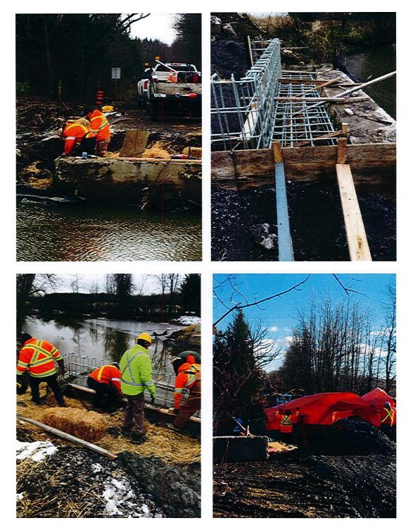
The concrete installation required significant rebar installation for the abutments. The concrete had to be completed in 2 pours; one for the base and another for the bearing
