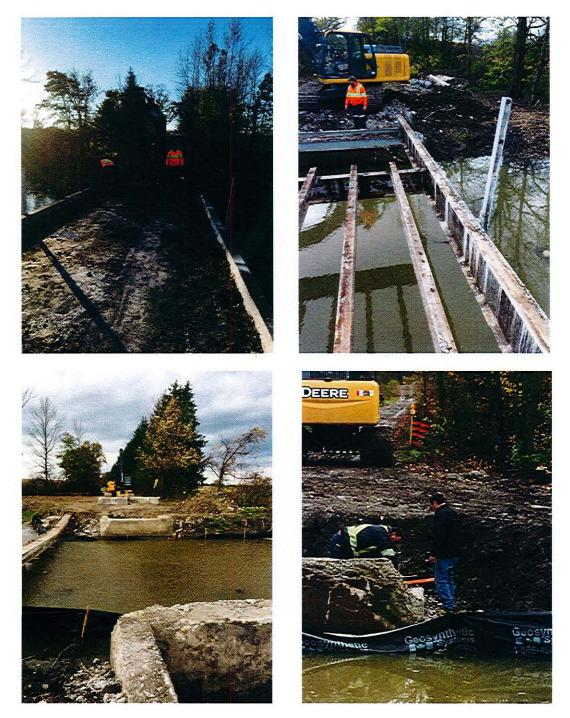
Removals of the structure consisted of the cutting and demolition of various concrete and steel appurtenances. The existing abutments were to be retained and new abutment constructed behind the existing to avoid in-water work.
