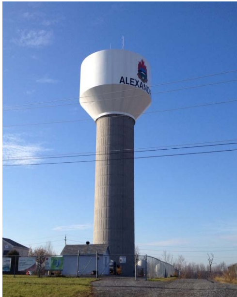
Photo 3-1 Alexandria Elevated Water Storage Tank
