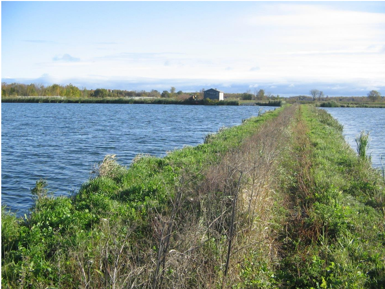
Figure 1-2– Alexandria Sewage Lagoon Facility
