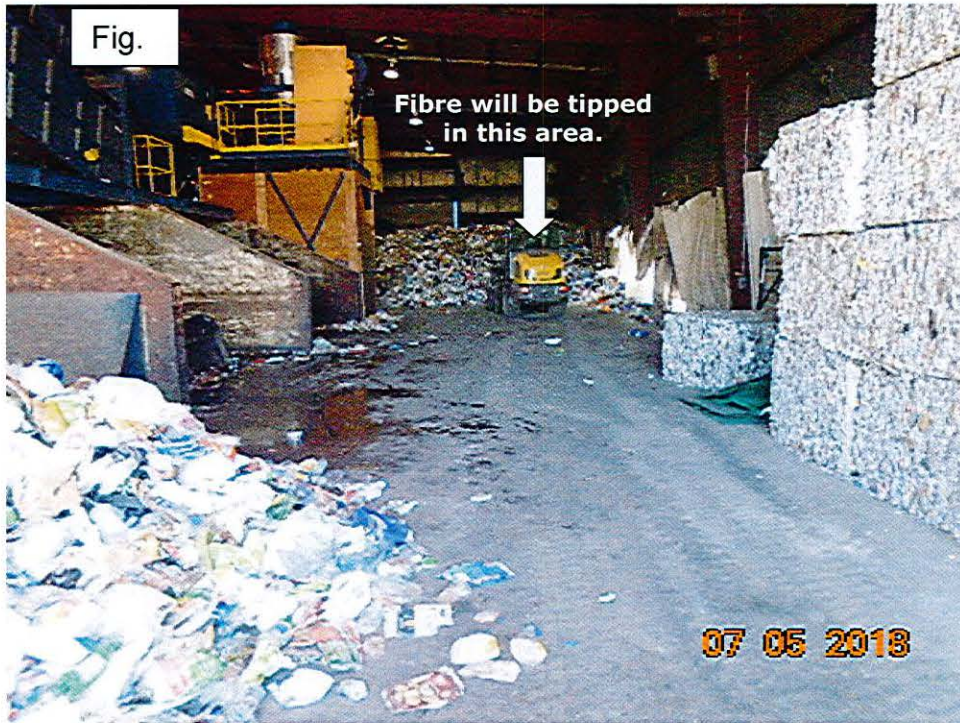
This is the old tipping floor, which was used before the installation of the equipment purchased in 2011. Tipped fibre will be fed to the HT Storage Unit (not seen in this photo) from inside the building.
