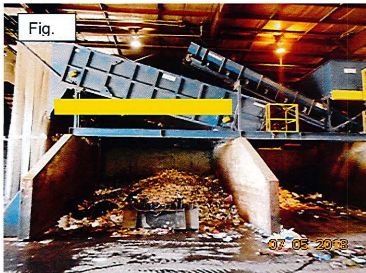
Yellow line shows the placement of the new sliding conveyor.
