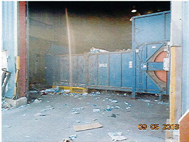
HT Storage Unit which is the start of the production line. It will be fed from this side for container sorting, and from the opposite side for fibre sorting.
