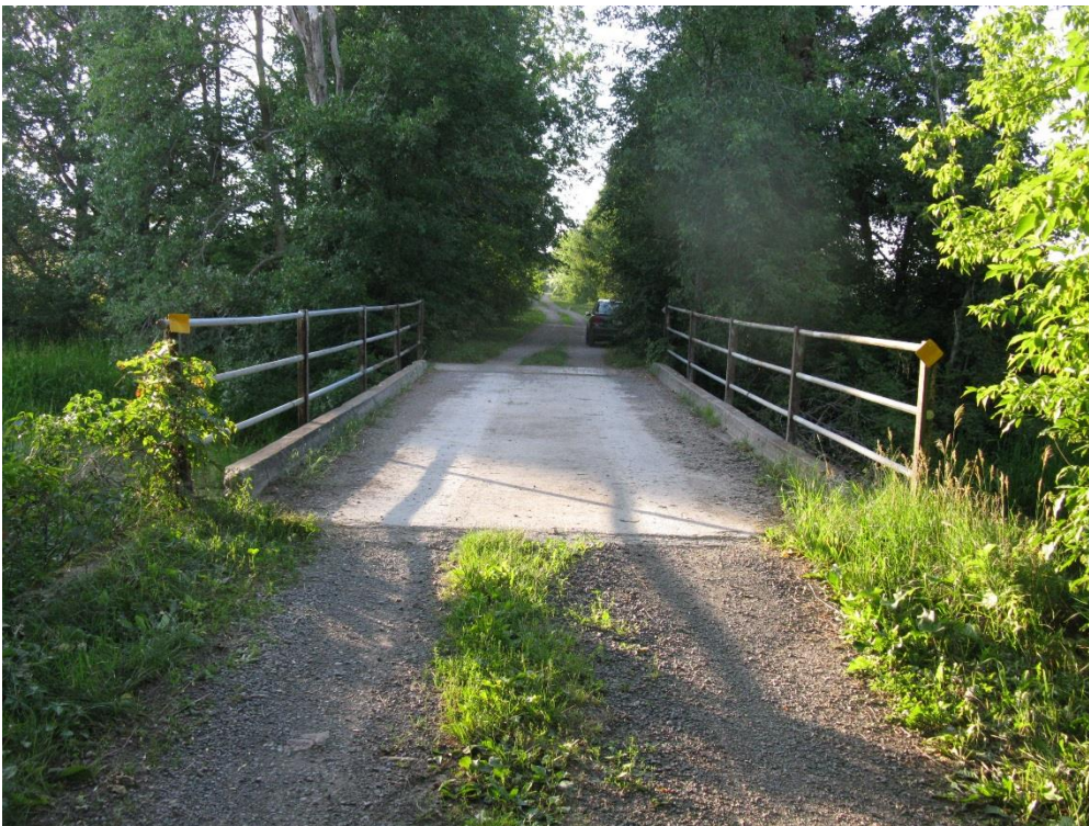
Picture 2. Overall view of top of the deck looking north.
