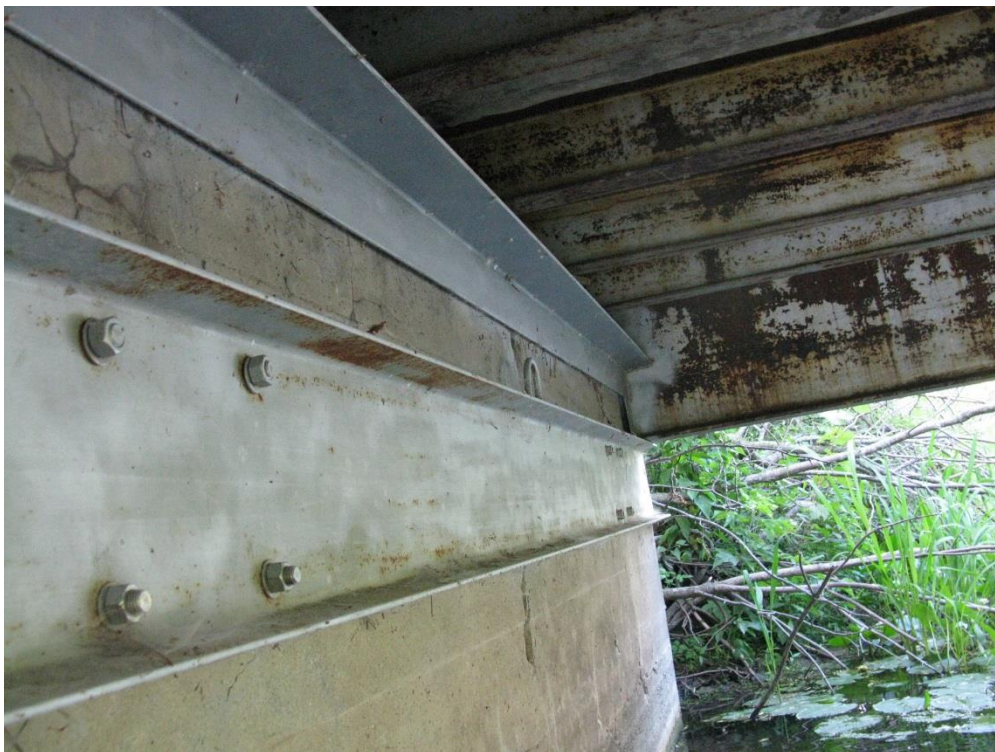
Picture 6. Steel channels were bolted to abutments to support the girders.
