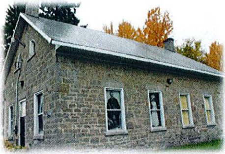
Kenyon Township Hall
