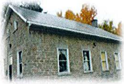
Kenyon Township Hall
