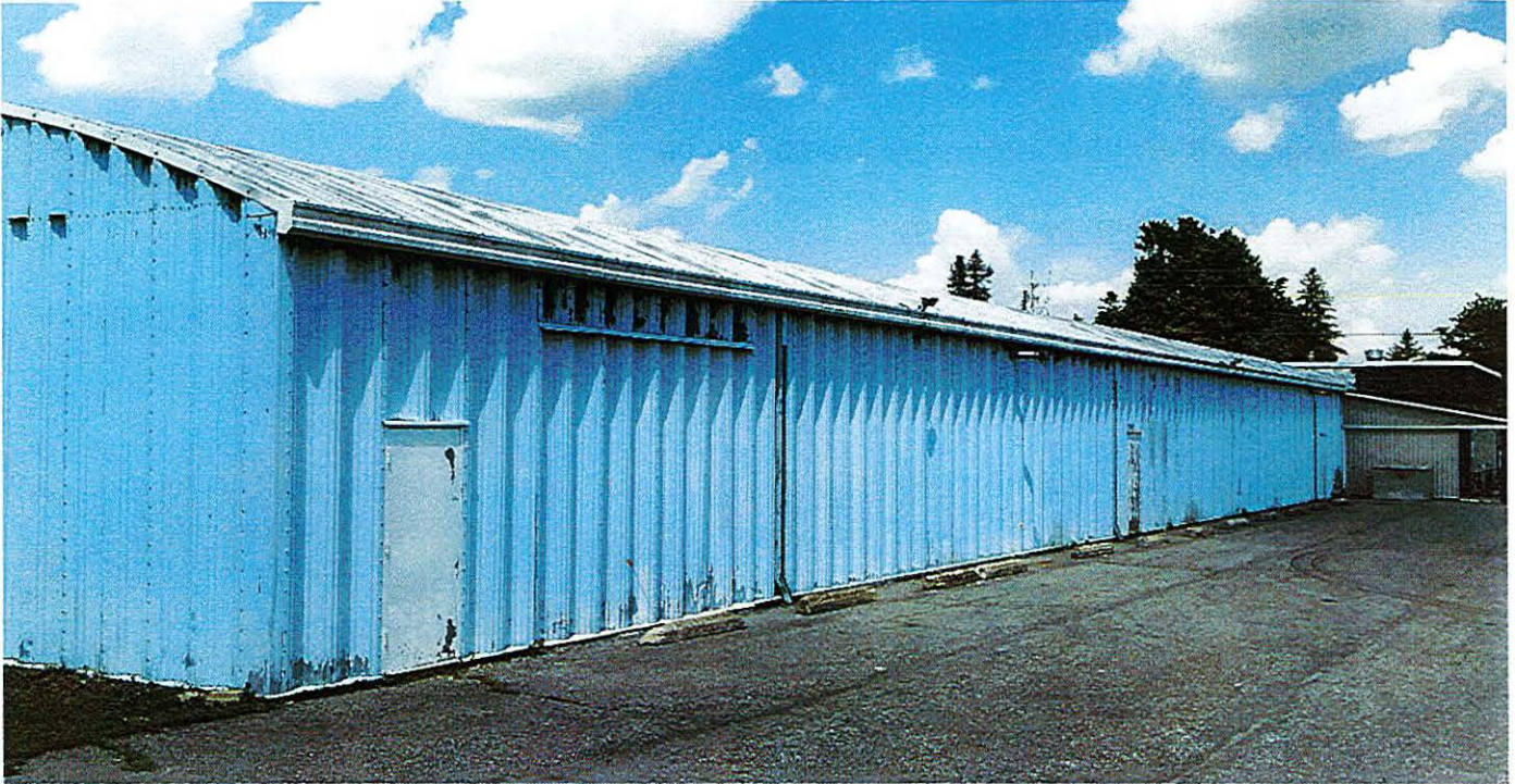
View of the West façade (looking towards Main Street)
