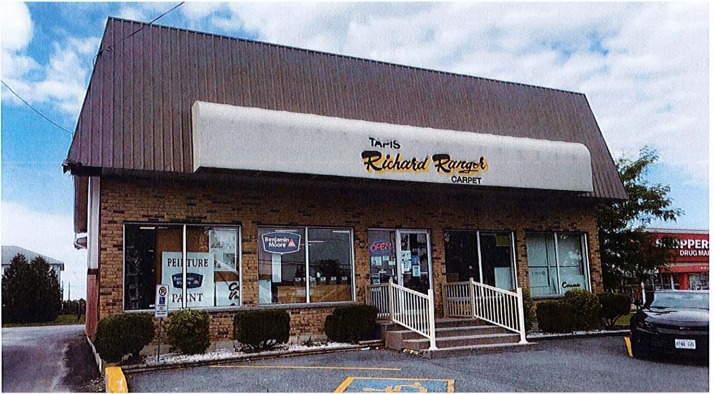
Photo of existing front façade
